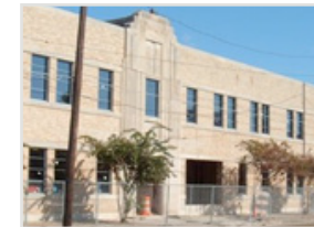
LeadX for office renovation American Red Cross Central Louisiana
