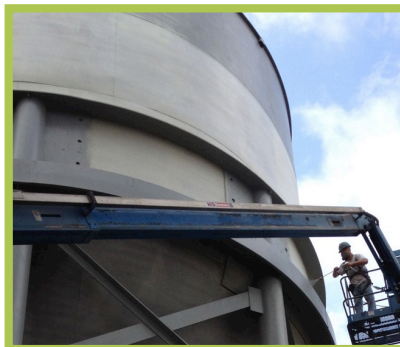
Tank Insulation Weyerhaeuser Pulp/Paper Savannah, Georgia, USA
