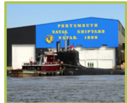
Metal Building Insulation & Protection U.S. Navy Portsmouth Naval Shipyard, Maine
