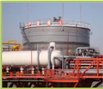
Insulation & CUI Mitigation Sinopec - Offshore East China Sea
