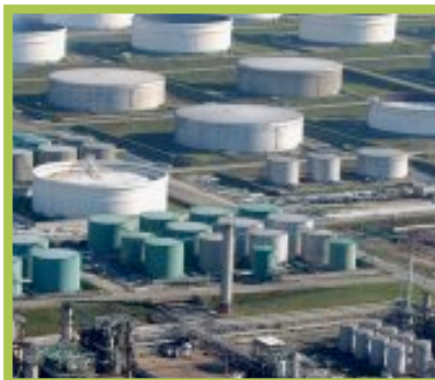
Pipeline & Storage Tank Insulation Galp Energia Portugal
