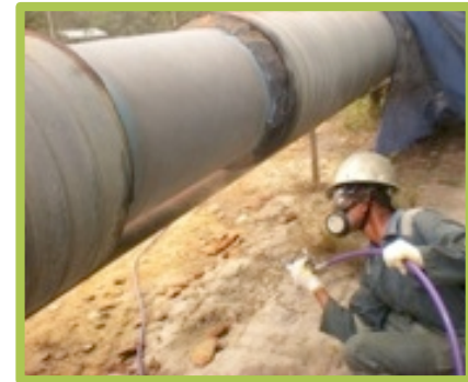
Insulation & Corrosion Control Hot Water Pipeline Indonesia
